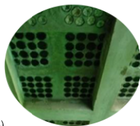
Filler slab with glass bottles.
