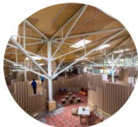
Roof is supported on eight columns in the form of a branching tree.
