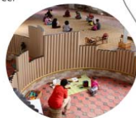
class room partition with paper tube
