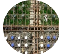
Filler slab with glass bottles.
