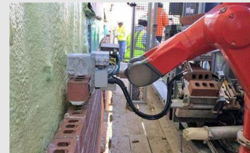
Brick laying Robot
