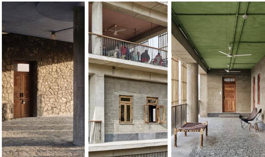
Figure 3-16 Refurbished and Re-used material
