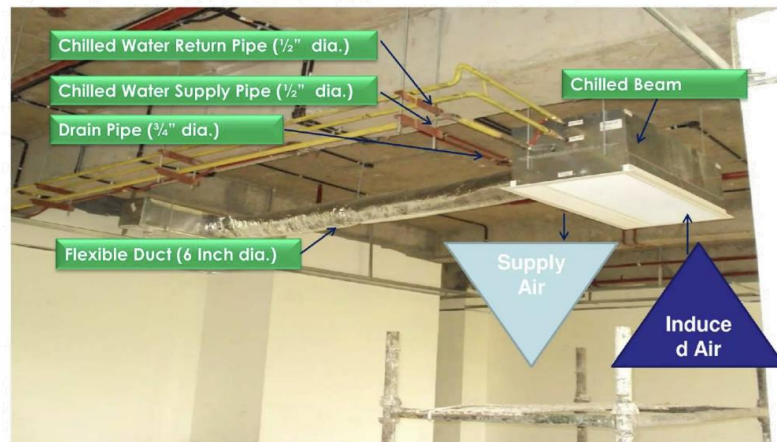
Figure 3-27 Chilled Beam Layout
