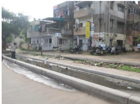
No stormwater run-offs
