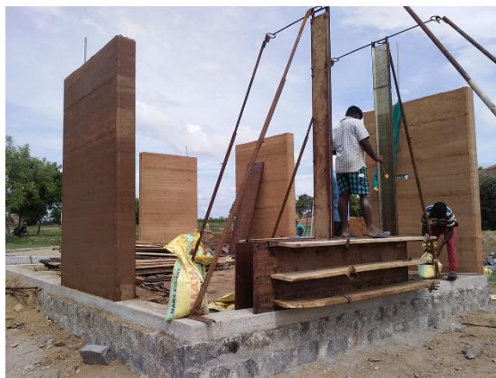
Fig 3.2 : Construction of rammed earth
