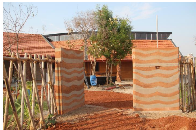
Fig 3.2 : Construction of rammed earth
