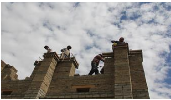
Fig. 6.29 Finishing of walls
