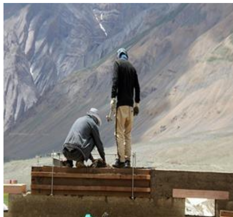
Fig.6.32 Rammed Earth Walls
