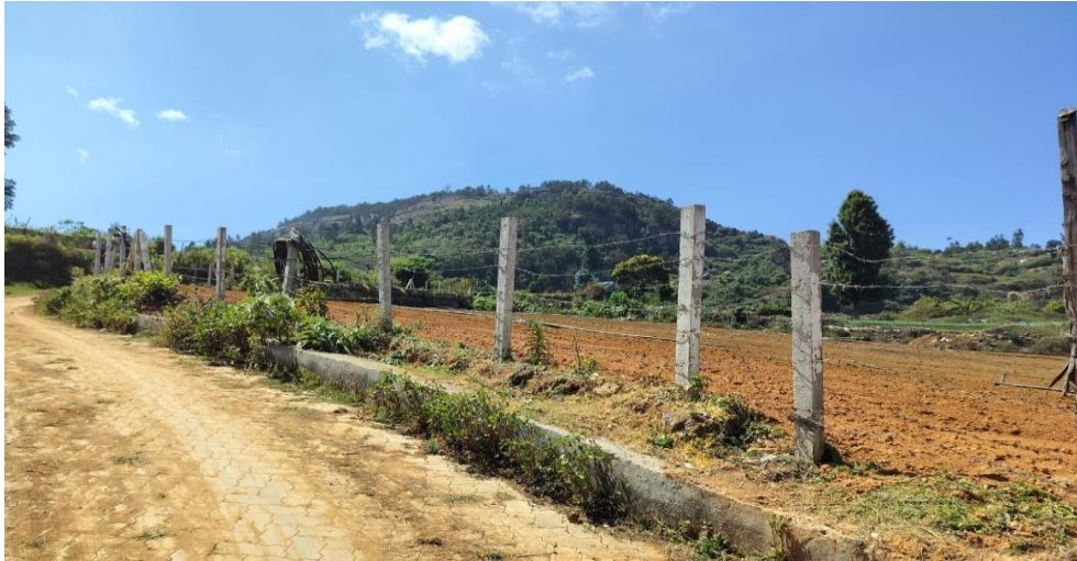
Fencing around the site
