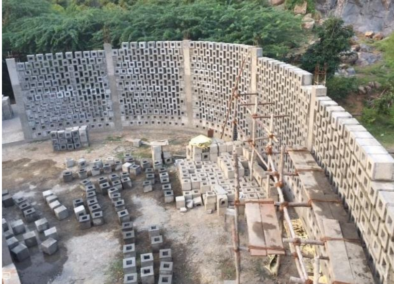
Fig.6.55 Construction of the community center
