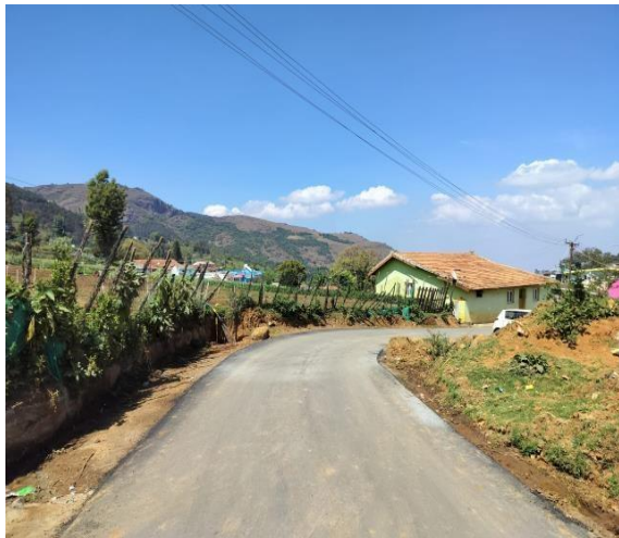
Concrete 4m Roads
