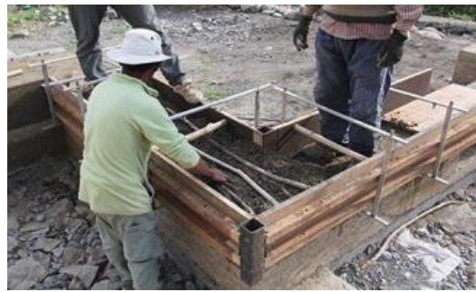
Fig. 6.30 Reinforcing the corner
