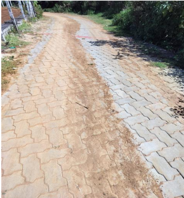
Paver block 3m Road
