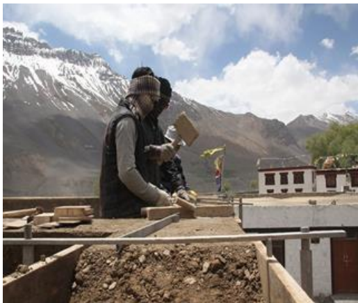
Fig.6.31 Traditional Ramming technique
