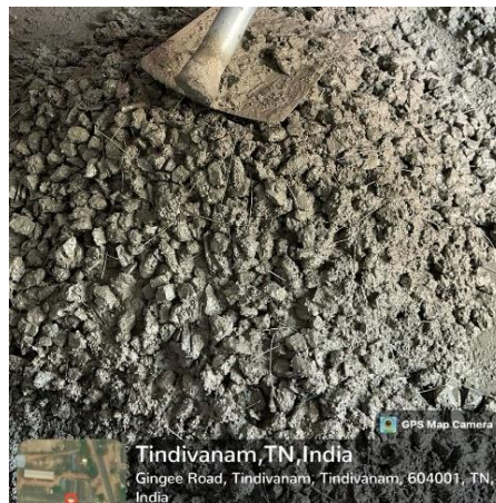
Figure 3.8: Mixing of concrete
