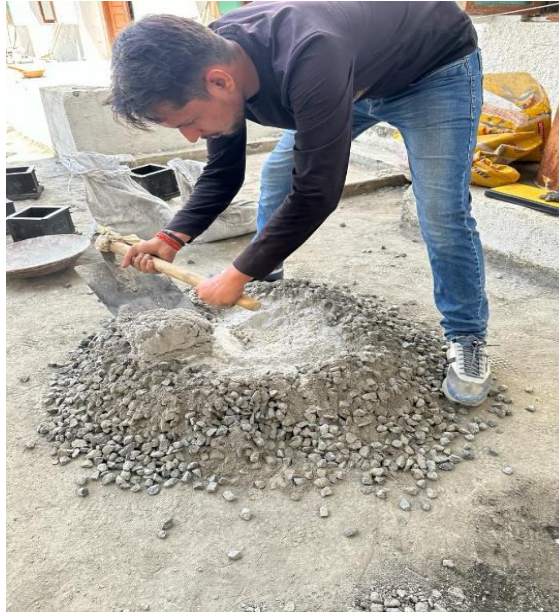
Fig 4.5: Hand Mixing of a Fresh Concrete
