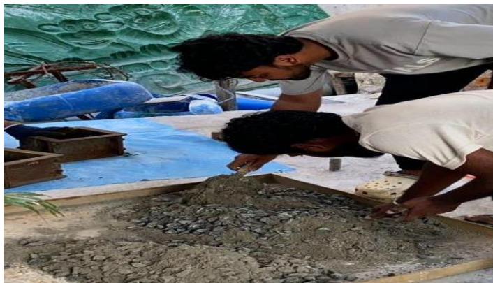
FIG 4.6 Mixing of concrete
