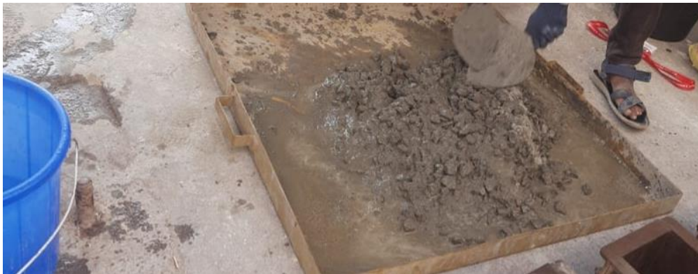
Fig 4.2 Preparation of concrete
