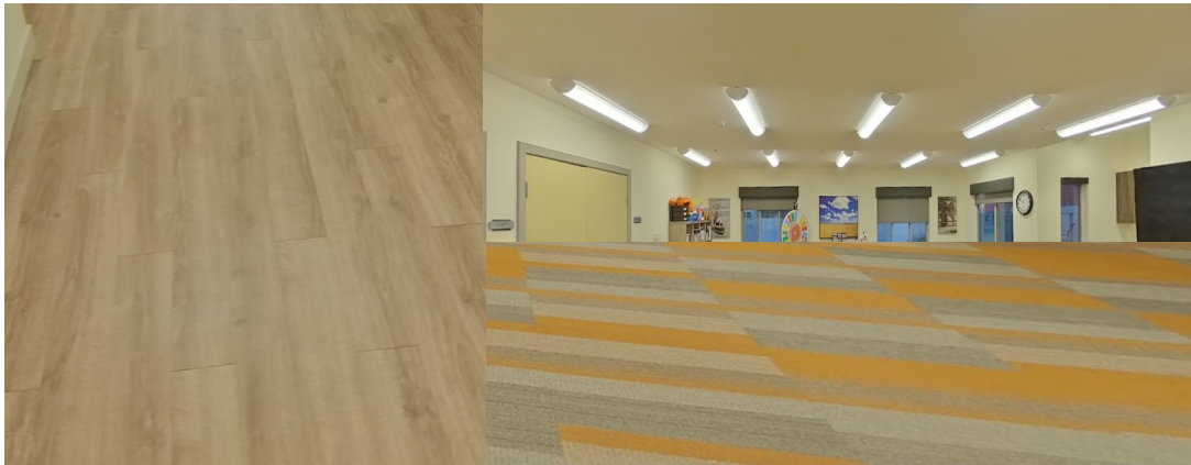
Fig 3.2 - Vinyl floor , LED rectangular light and carpet flooring
