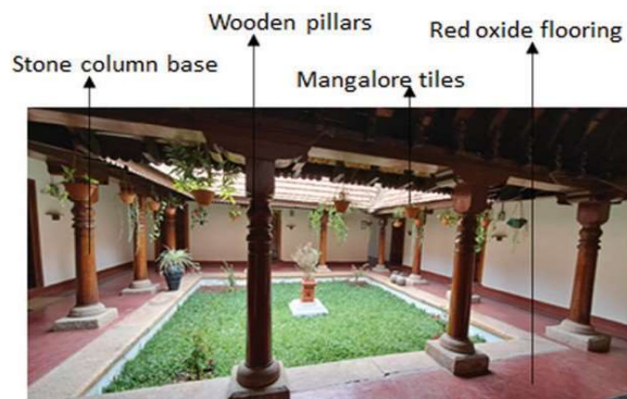
Figure 19 Material used in the Building
