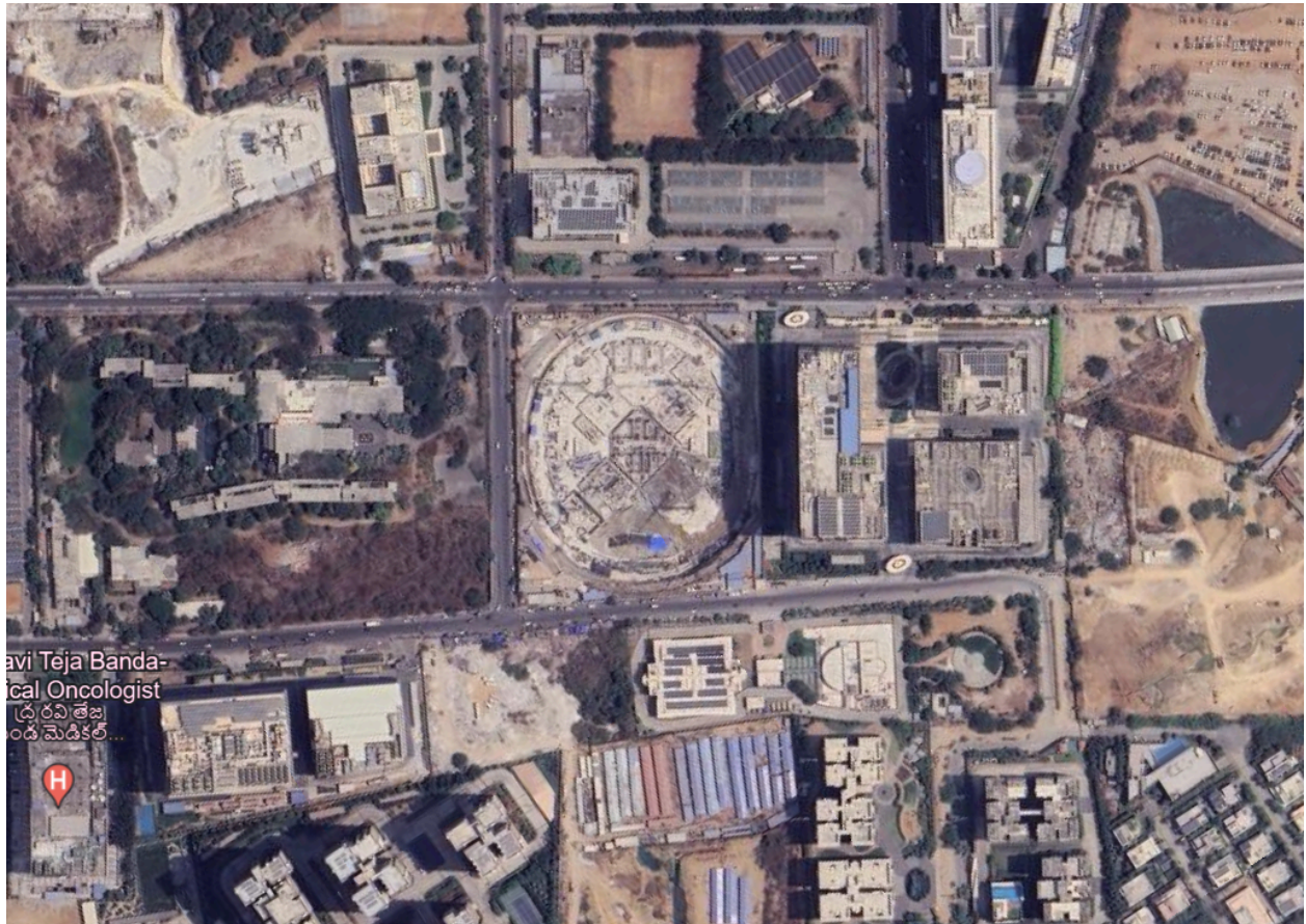
Fig 5.1: Site from google earth
