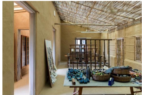
Figure 2.11: Designer studio to create diffused light and semitransparent bamboo roof
