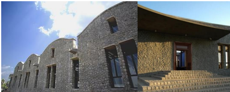
Figure 2.19: The exterior views of the building which shows the intense Rubber Mansory Wall, source: SJK Architects
