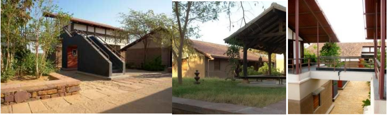
Figure 2.41: The Pause points in between building clusters, Overhead walkways connect the upper floor level
