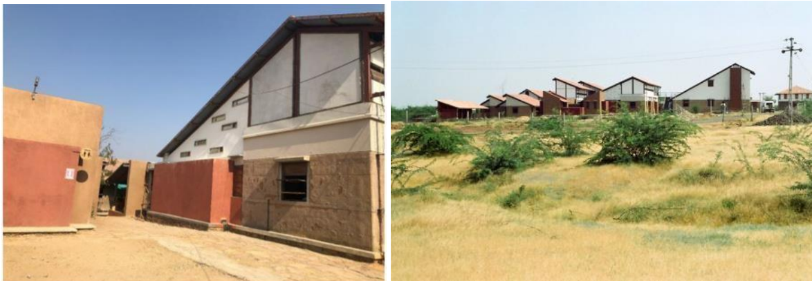
Figure 2.42: The workshop area and overall block view facing the rear side of the site
