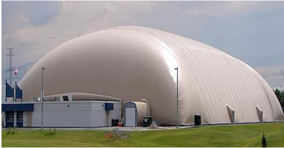
Air Supported Structures
