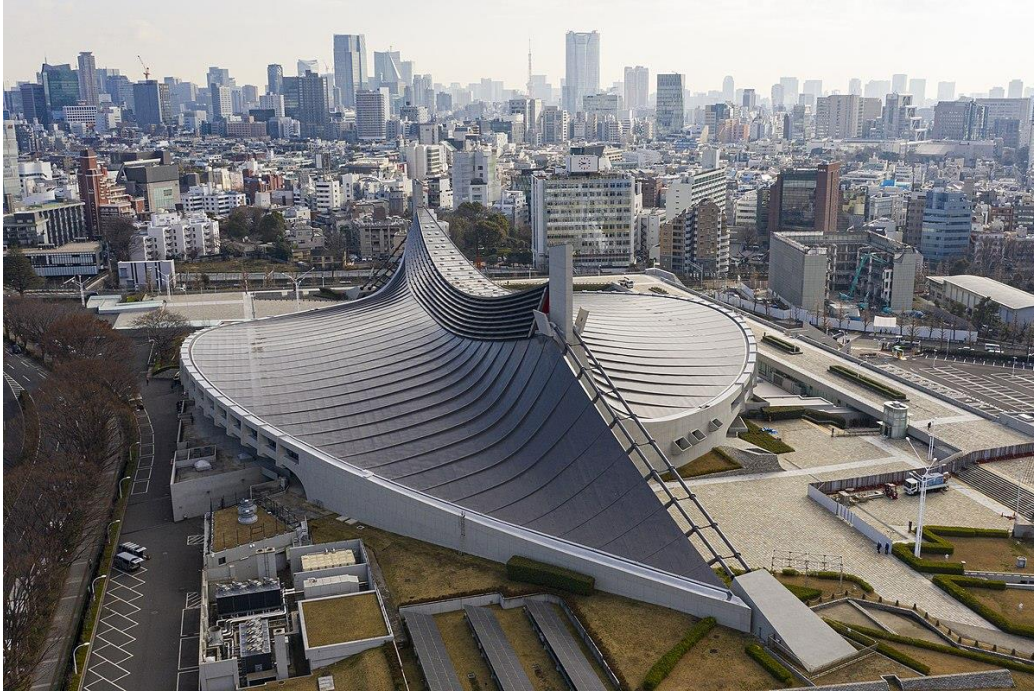
Figure 9 Yoyogi National Gymnasium
