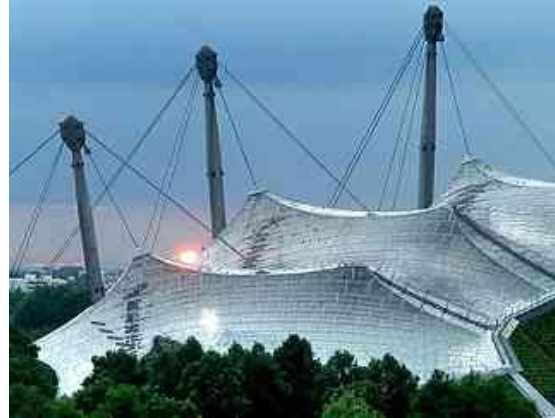
Cable Stayed Roof
