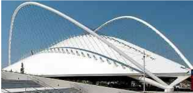
Cable Suspended Roof
