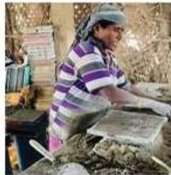
Step 5: Laying the wet mixture
