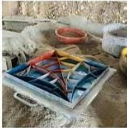
Step 1: Placing the mould over the glass which is fitted into the frame
