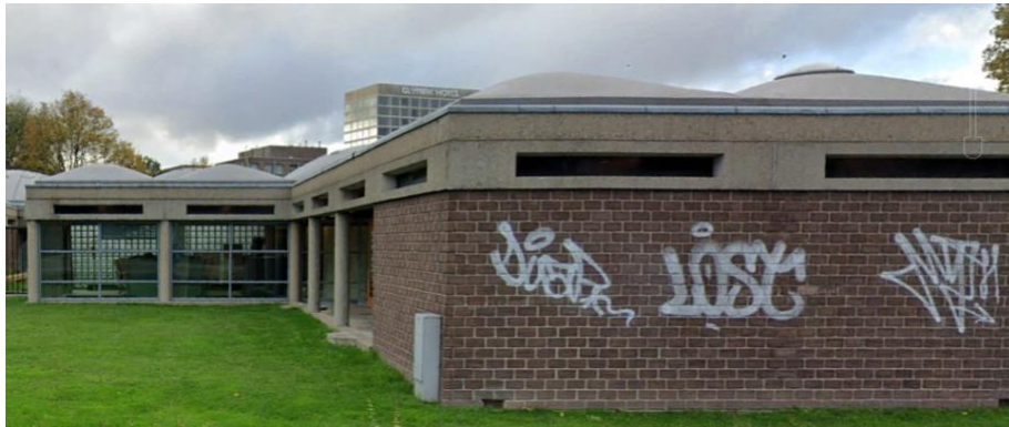
Fig 3.5: Brick wall material
