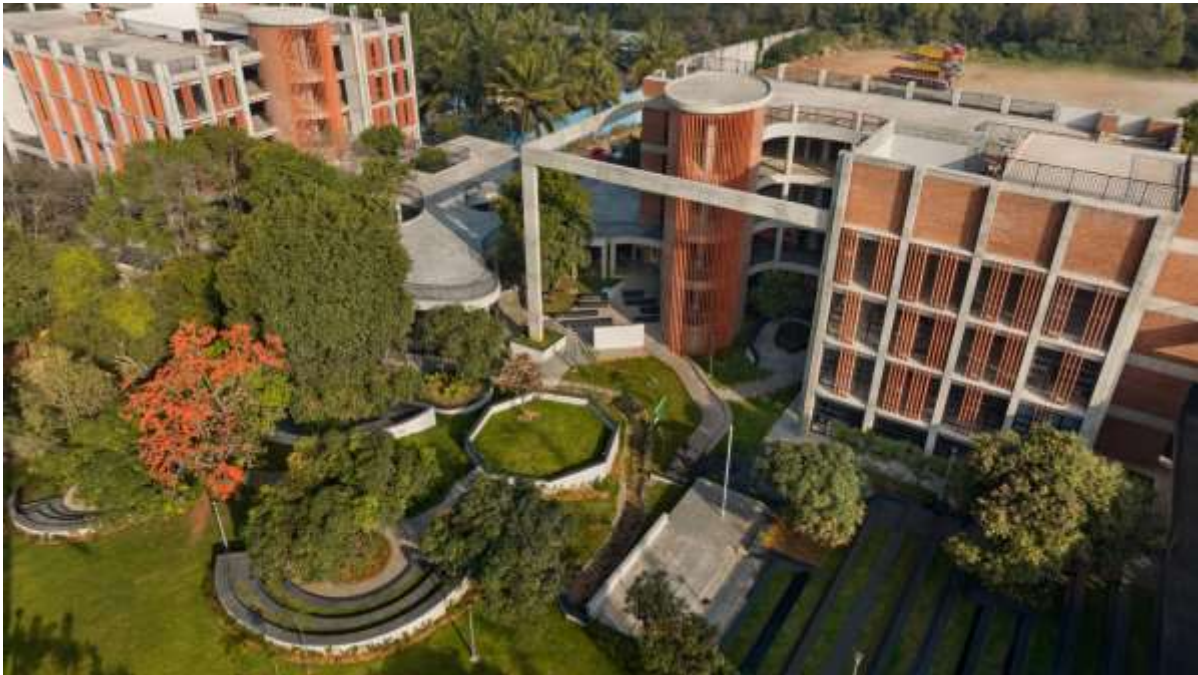
Figure 2.10 Academic Block. Image Source : (Vijay Gupta Architects)
