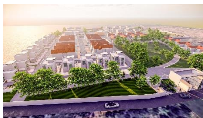
Fig: 8.2 Overall view 1
