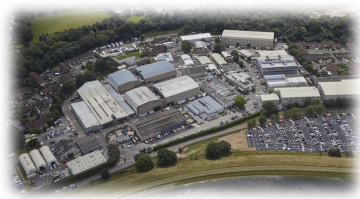
Fig 2.5: Aerial view of pinewood studio
