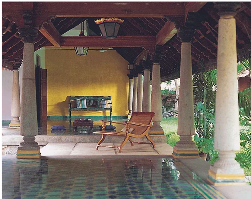
Figure 5.2 Chettinad columns, Athangudi tiles and granite stone along the edges, eave boards, timber rafters etc. add character to the house.
