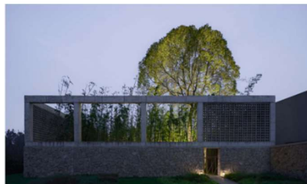
Figure 2.18 Image of exterior
