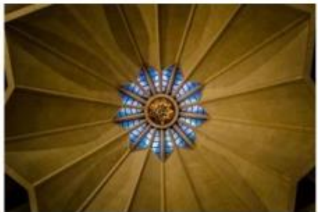
Figure 3.28 Steel and glass roof skylight
