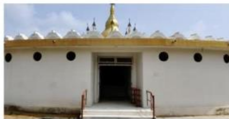
Figure 3.57 Entrance of Pagoda complex
