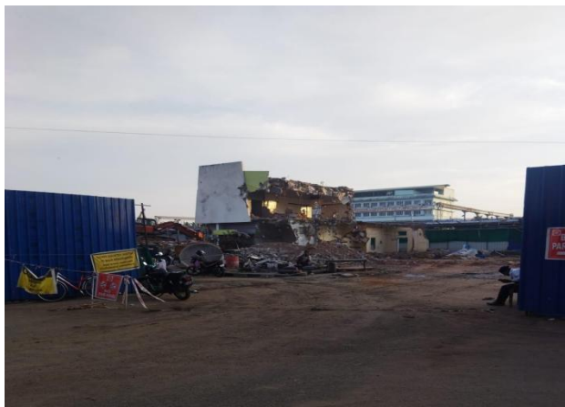
Fig 3.2: On going works
