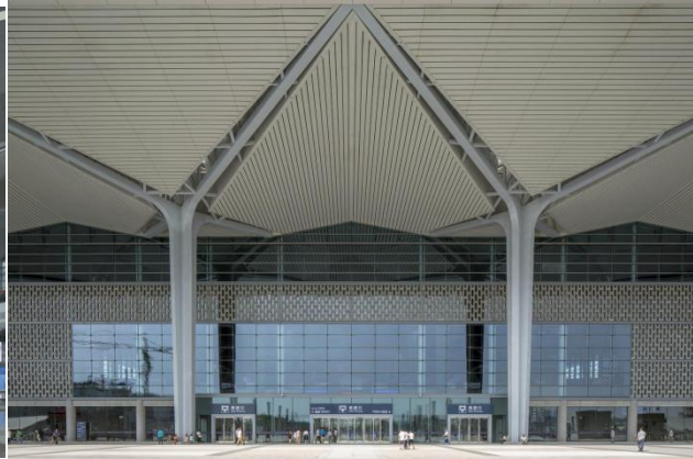
Figure 2.48: Support structure in the eastern side
