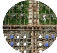
Filler slab with glass bottles,
