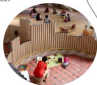
class room partition with paper tube
