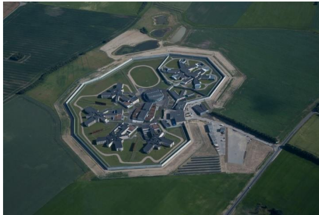
Figure 36-Aerial view of Storstorm Prison
