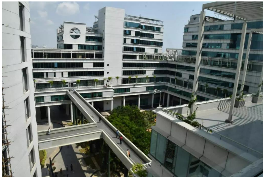
Figure 7: Connecting Bridge between towers A, D & E
