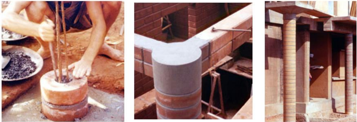
Figure 6 - composite column types details(earth-auroville.com)
