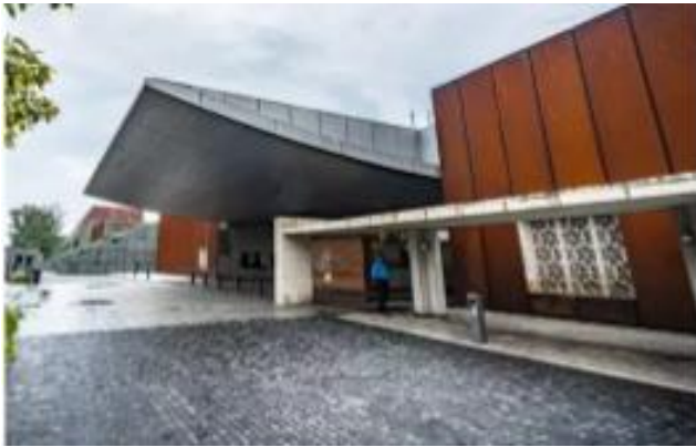
Fig 2.29(a): Weathering steel in Foyer Projection Fig 2.29(b): Eps insulation in wall
