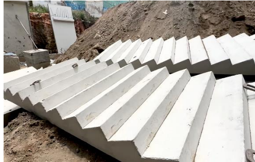
Figure 6.6 Precast concrete stairs
