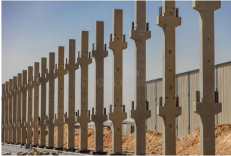
Figure 6.4 Precast columns
