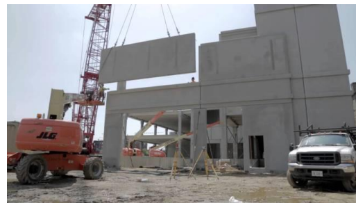
Figure 6.3 Fixing of wall panel
