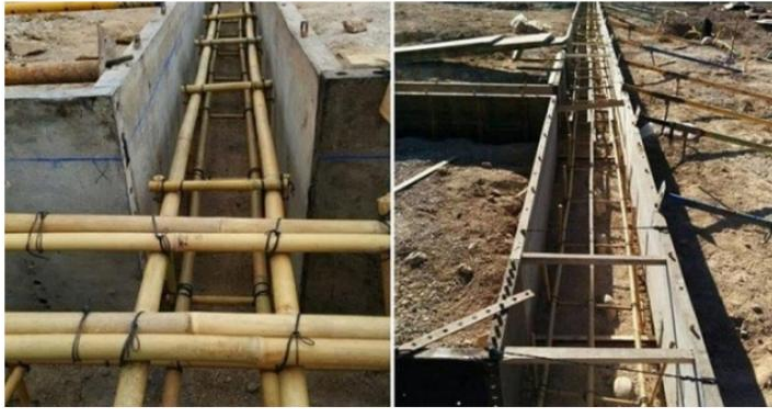
Fig 4.6: Bamboo in Foundation
