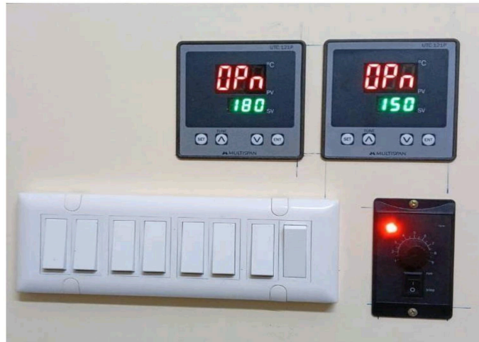
Figure 4.15: Motor Speed Controller
