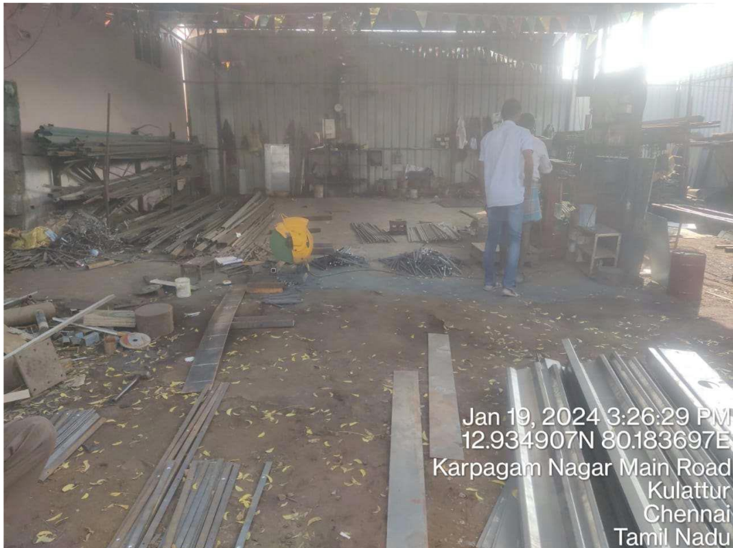
Fig 3.3 welding of corrugated beam
