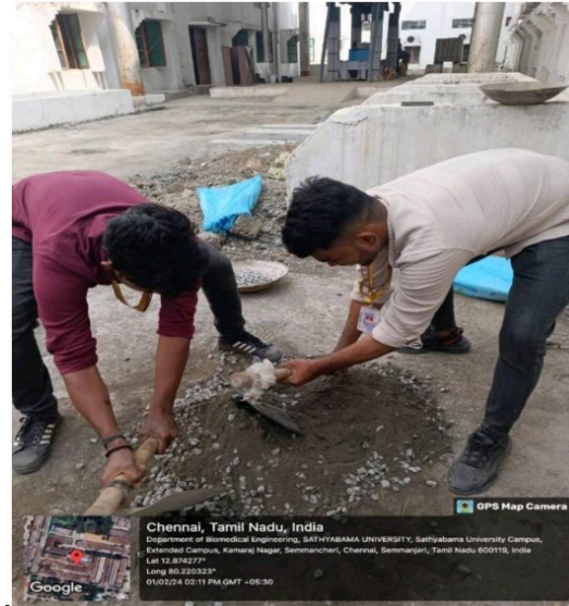
Fig: 4.6: Casting of Concrete
