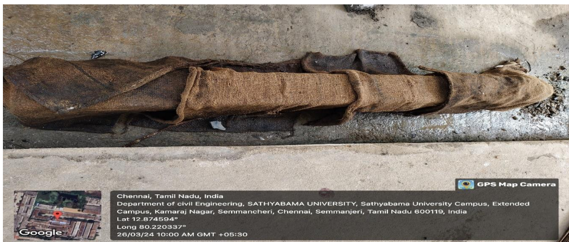
Fig 4.5 After Removal of Shuttering Plates
