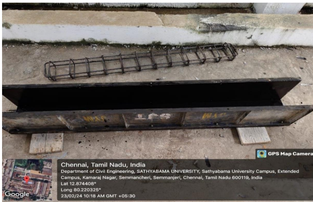
Fig 4.3 Shuttering Plates for Beam Casting
