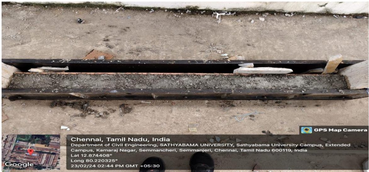
Fig 4.4 Casting of Beam
