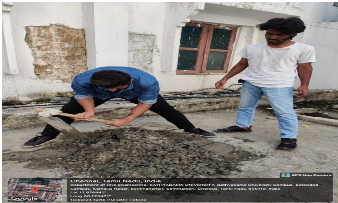
Fig:4.1 Mixing of Concrete
