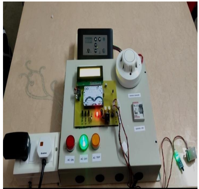
Fig. 7 AC controller switched ON
