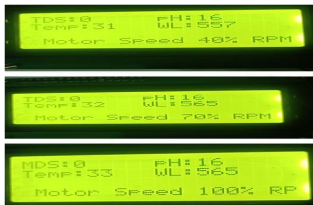
Figure 16: LCD Display for Fan Speed Control Based on Sump Water Temperature
