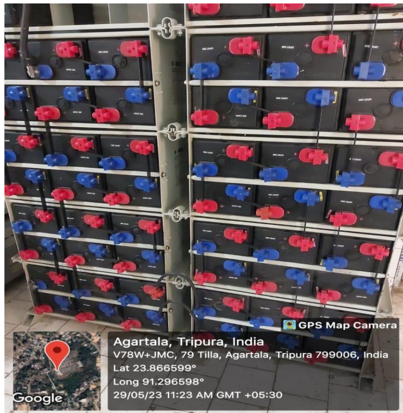
Fig: 110V Battery Bank
