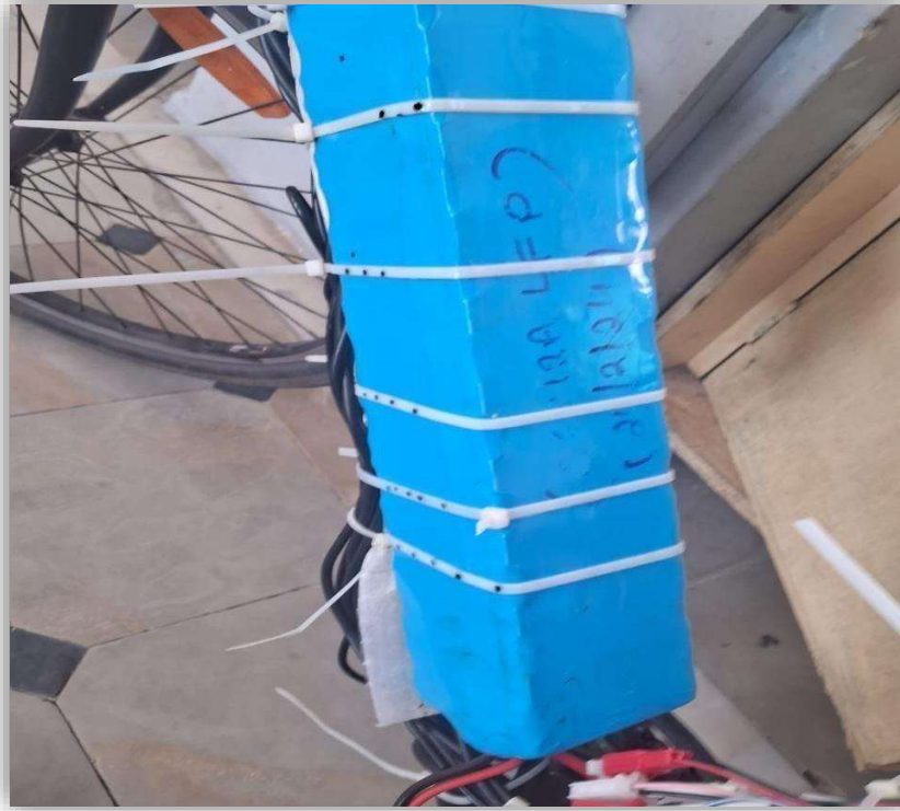
Figure 6.3 After installing the battery
