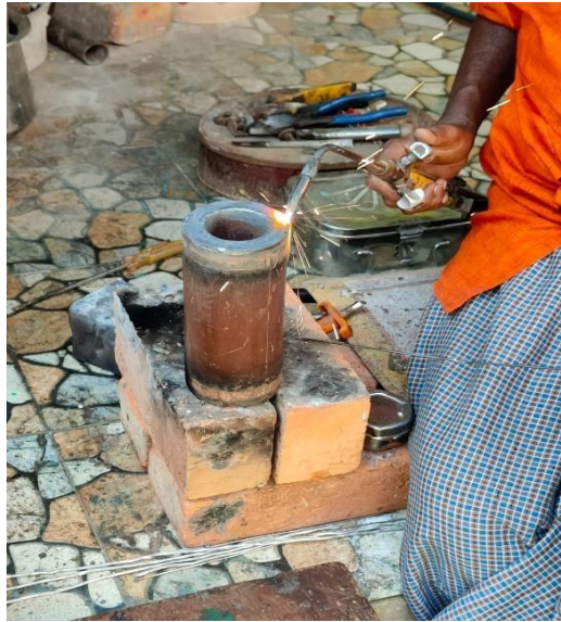
Fig:4.2 : Welding of Combustion Chamber
