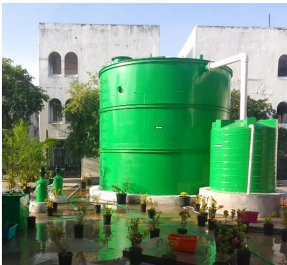
1 Tonne capacity Biogas Plant converts Food Waste generated in the Institution Mess to Biogas replacing 3 commercial cylinders daily
