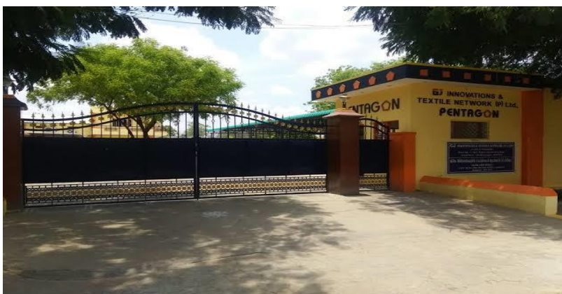
Fig 1 Front view of the company
