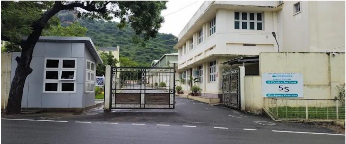
Fig 2(Front view of the company)
