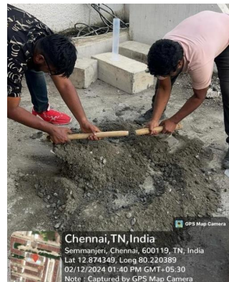
Fig 5.2: Mixing of Concrete Mix
