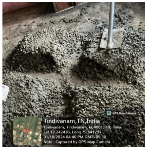
Figure 3.7: Volume batching
