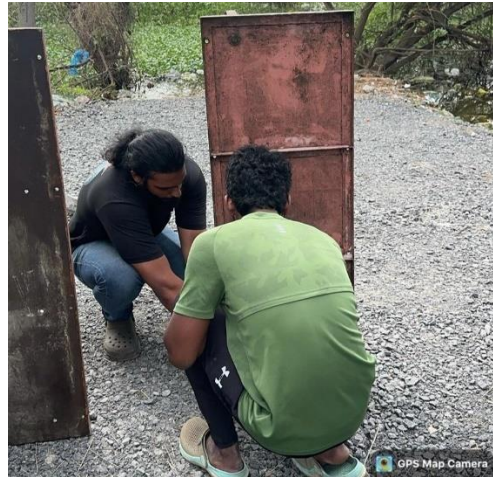
Figure 3.6: Preparation of mould
