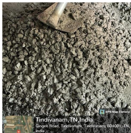
Figure 3.8: Mixing of concrete
