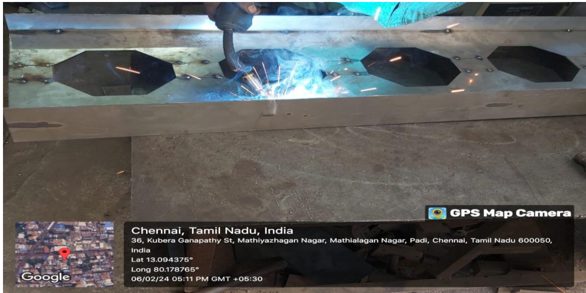
Fig 3.6: Welding of Beams
