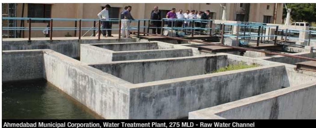
Ahmedabad Municipal Corporation, Water Treatment Plant, 275 MLD - Raw Water Channel
