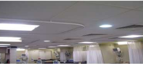
Stainless steel ceiling
