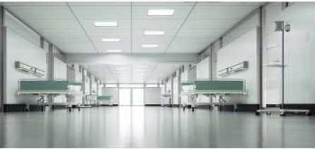
PVC false ceiling
