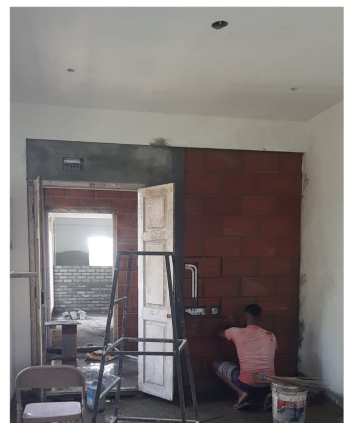
•Salvaged doors repaired and used for all maindoors of the units
