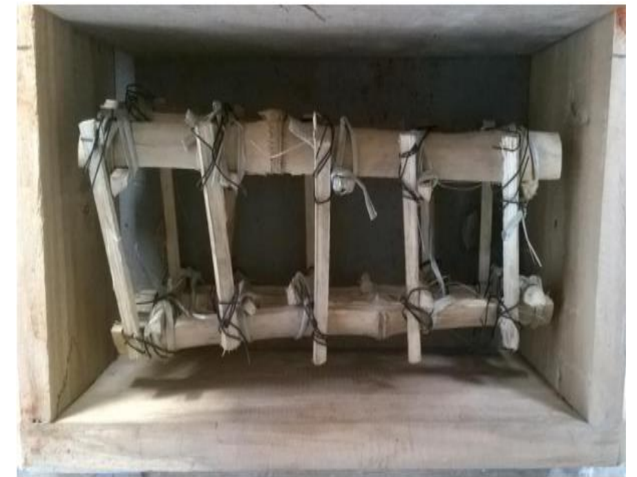
Formwork placed inside the mould
