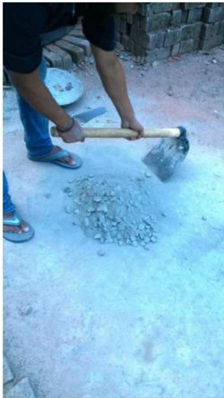
Mixing of cement concrete
