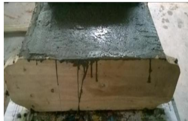
Concrete placed in the mould
