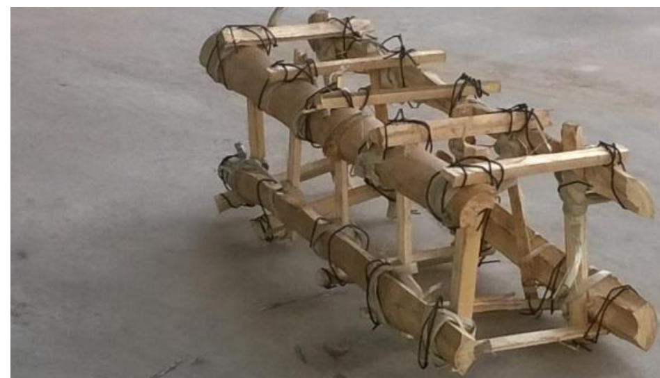
Formwork of bamboo reinforcement(2 layers)
