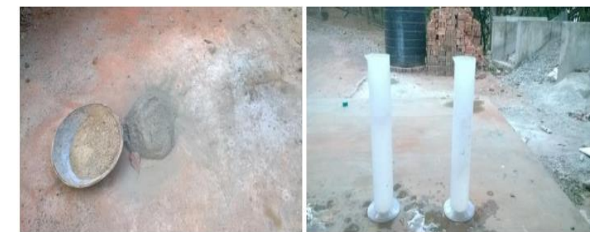
Volume batching of M20 cement grade
