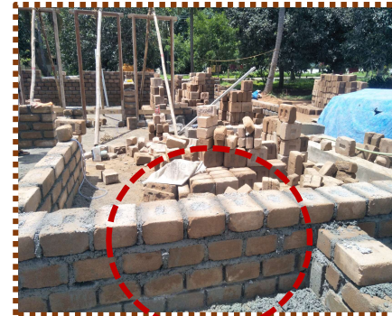
The binding of the blocks using the soil & cement.....
