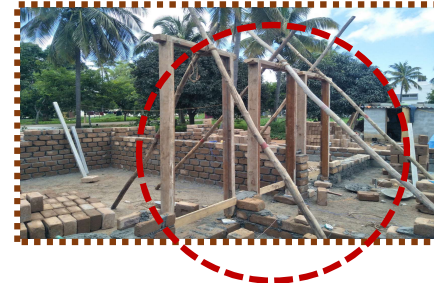
The upcycled door frames & wood from the old dilapidated projects.....
