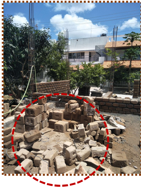
The CSEB blocks of 300 mm thickness for the walls....
