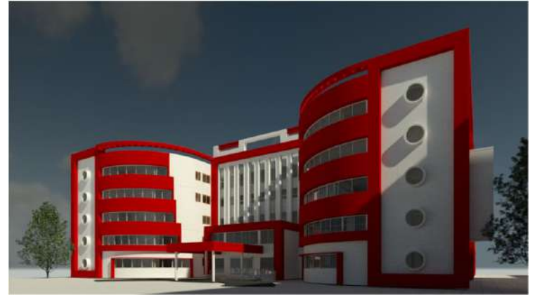
FIG 04: NORTH – FRONT VIEW
