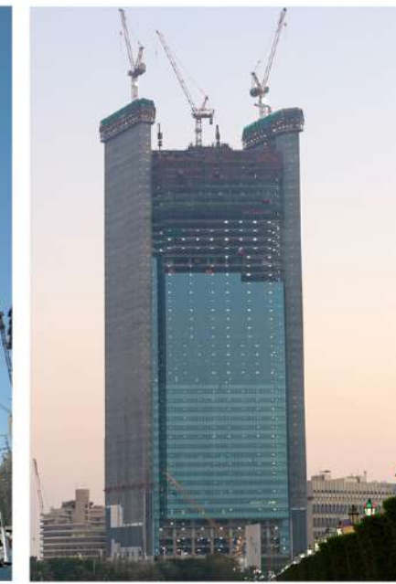
ADNOC HEADQUARTERS, ABU DHABI
