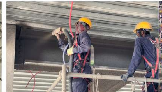
CEMENTITIOUS SPRAY FIRE-PROOFING OF 20 mm
