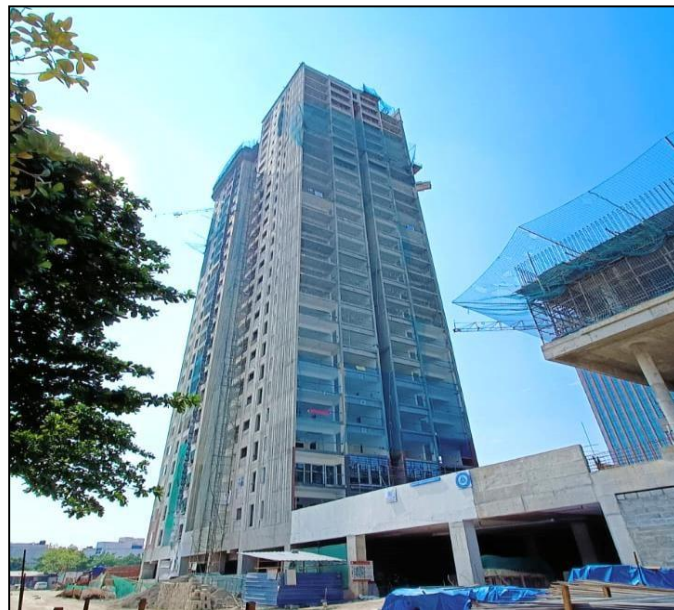
TERRACE SLAB IN PROGRESS
